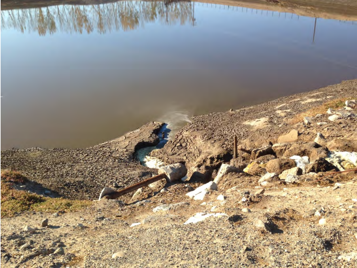
Photo: View to southwest of Lagoon 1. Dried, cracked, and eroded manure seal is visible in foreground.
