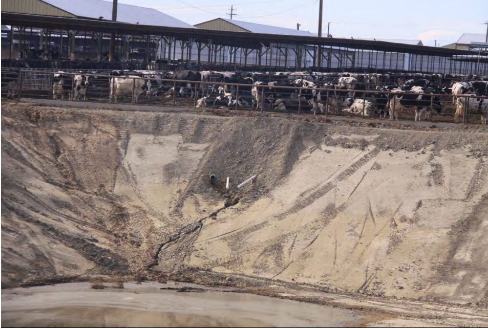
Photo. View of NW Catchment Basin during October site visit. New liner with significant erosion from infall pipes is shown
