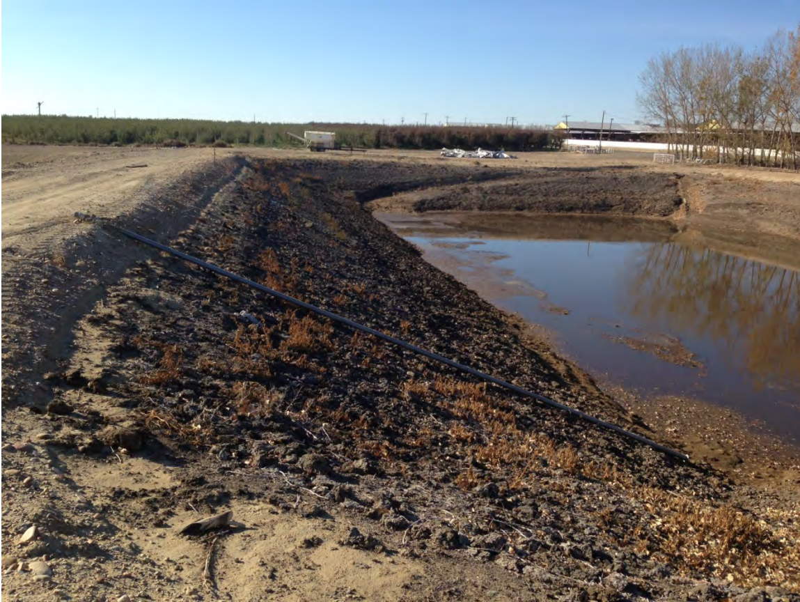
Photo: View to the west of Lagoon 2. Dried and cracked manure seal on sloped sides of lagoon is visible on south end of lagoon.
