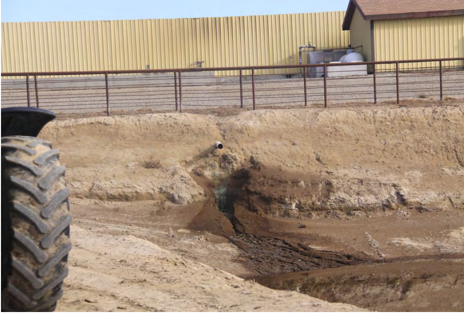
Photo. View of NE Catchment Basin. Note erosion from inflow and lack of manure seal.
